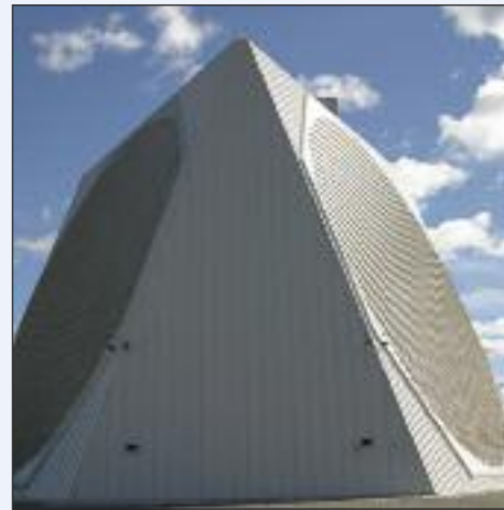
SSPARS Radar Clear Air Station. A Solid-State Phased Array Radar System radar in a protective dome stands 11 stories tall on Clear Air Force Station. The station's primary duty is to provide an early warning of intercontinental ballistic missiles and submarine-launched ballistic missiles.
